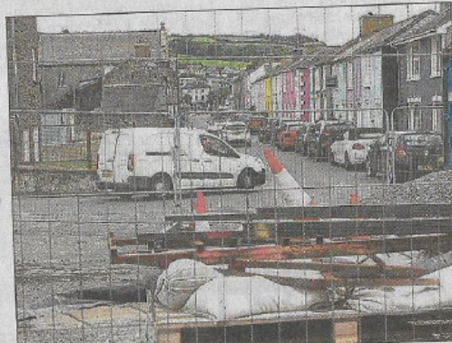
The closed car park on Tabernacle Street.
